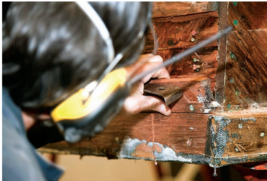
Much of the boat's 3/8-inch mahogany planking had to be replaced.
